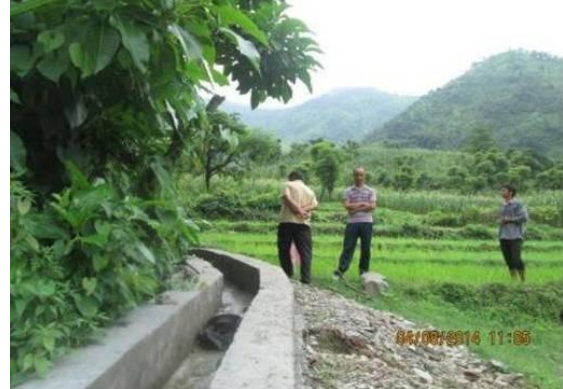
SPMP support -Irrigation canal at Dattu VDC, Darchula district
