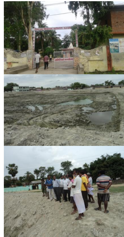
1. Dhanusa DDC premises, 2. Ongoing pond management in Baniniya VDC and 3. On site inspection of Pond conservation work in Baniniya
